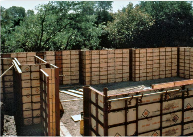
The Steel-Ply forming system is a pre-engineered, factory-built, reusable concrete forming system. It may be used in handset or gang form applications, for commercial or residential structures. The Steel-Ply forming system can form walls of almost any shape or size, with accessories for special structures and details. This system is more productive and economical than job-built plywood formwork or other forming methods.
