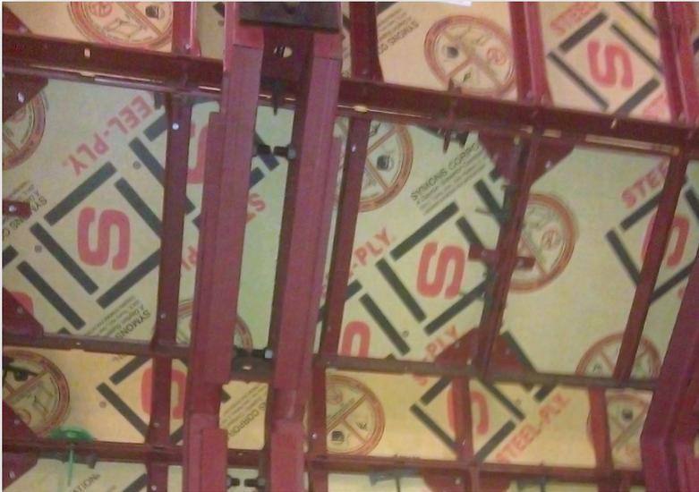
The most economical and productive way to gangform with Steel-Ply forming system is to use the load-gathering technique. Steel walers and strongbacks “gather” the load of the panels and high-capacity ties are installed through the panels and Walers. The load is transferred to the ties from the walers.
